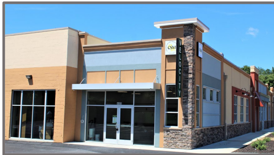
College of Southern Maryland, Velocity Center $274,000
